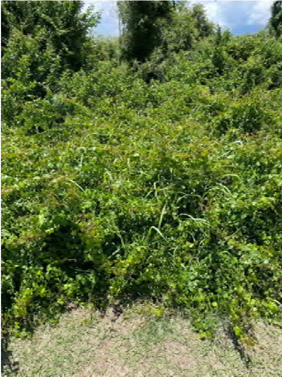
Location 15: Clear 6' access path and remove sediment/vegetation within 6' radius around end treatment to provide positive discharge of stormwater.
