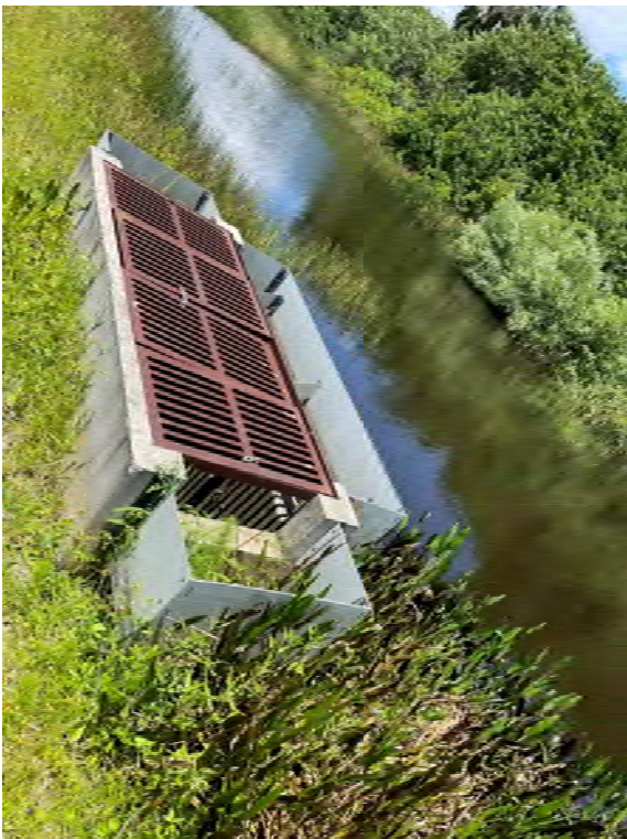
Location 16: Remove vegetation inside and within a 6' radius around skimmers.
