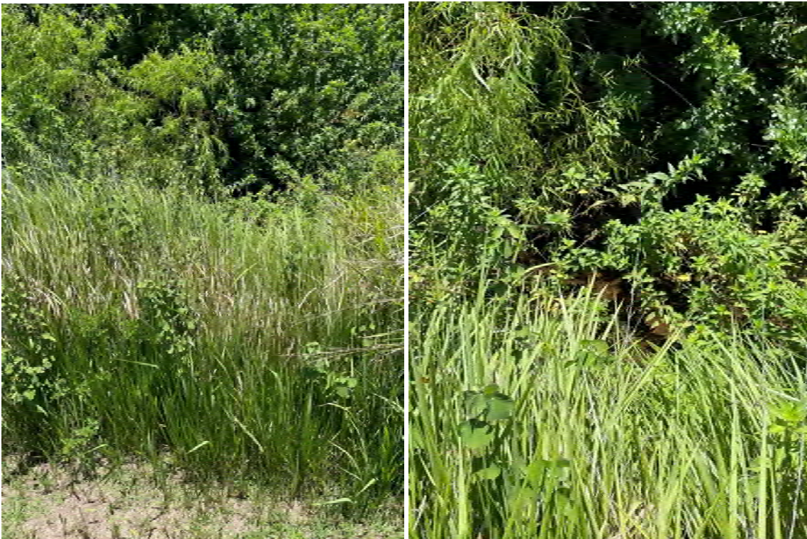
Location 10: Clear 6' access path and remove sediment/vegetation within 6' radius around end treatment to provide positive discharge of stormwater.
