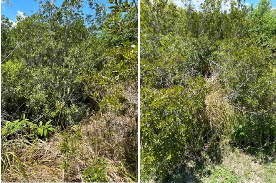
Location 9: Clear 6' access path and remove vegetation within 6' radius around control structure.
