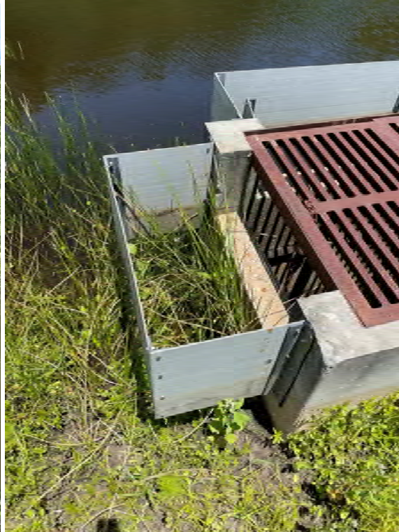
Location 16: Remove vegetation inside and within a 6' radius around skimmers.
